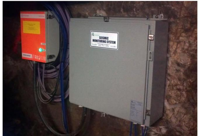
*Seismic monitoring system installed in an underground mine*
